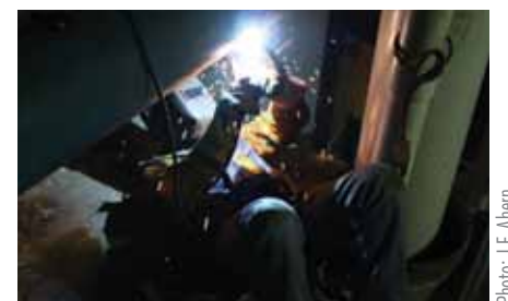
A welder at Schoeneck's Milwaukee facility.
