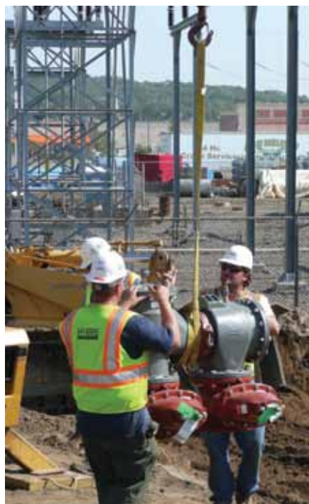
Contractors work on a commercial project.
