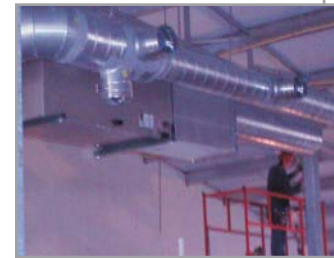
Installing ductwork at the North Metro Harness Racing Track.
