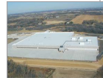
HiMEC is installing the Plumbing, Piping and Sheet Metal for the 475,000 sq ft. ALDI Project.
