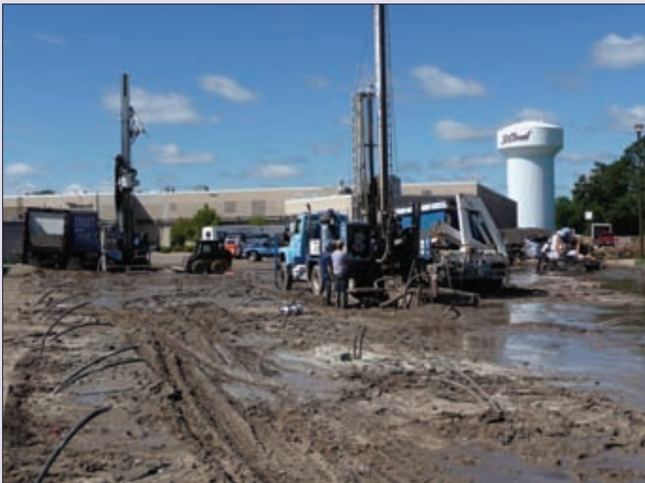
Contractors prepare for the GeoExchange well-field installation, adjacent to the MAC.
